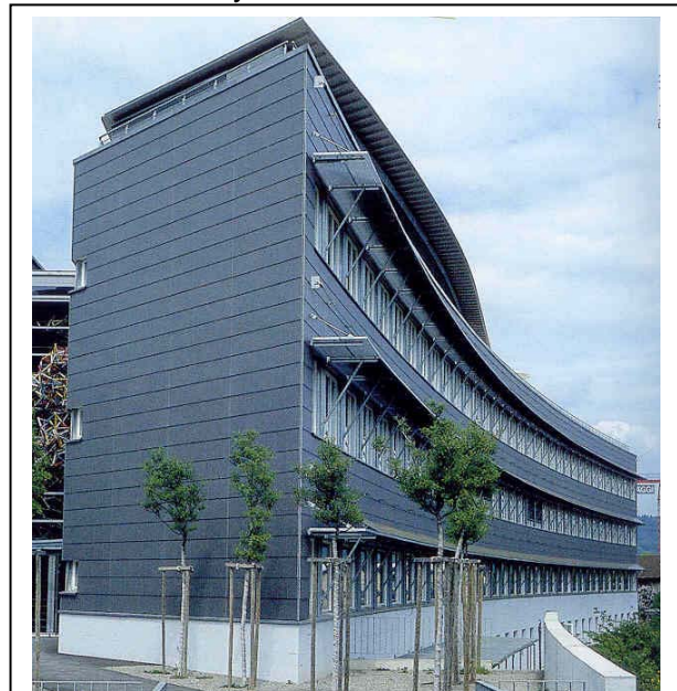
Window shade structure BIPV mounting technique
