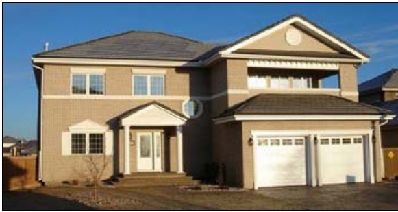
Non-rectangular roof surface - ETI Solar, Canada
