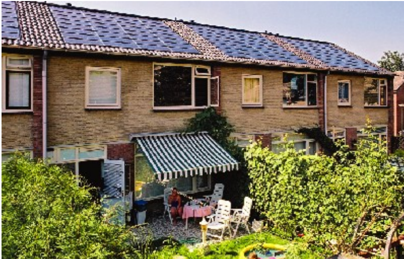
PV Installed on Attached Housing Units, Netherlands.
