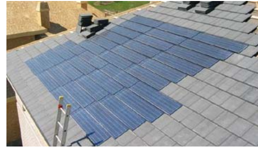
Close up of PV panels ETI Solar, Canada
