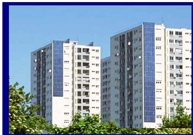
Figure 2 - 92 kWp Solar PV Community in France (source: ADEME)
